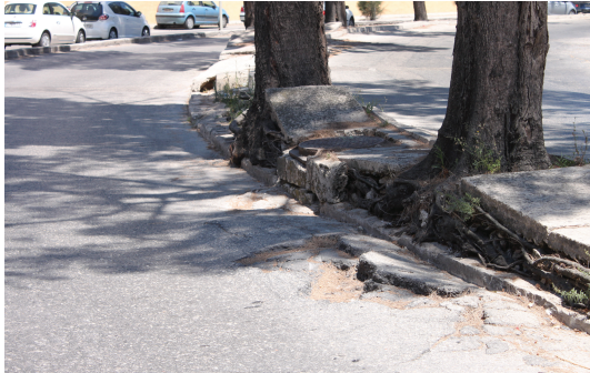
Figure 44. Damage to road by tree roots with safety implications
