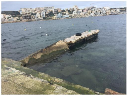
a number of fissures/voids have developed within the concrete structure, below sea level, making it more prone to an accelerated damage by the rigorous wave impact.
