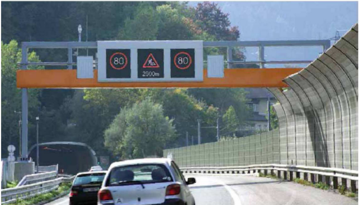
Figure 22: Example of dynamic line control road signs at the A12/A13 motorway in Tyrol
