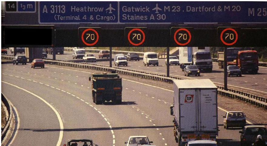
Figure 21: VSL system on motorway in the UK
