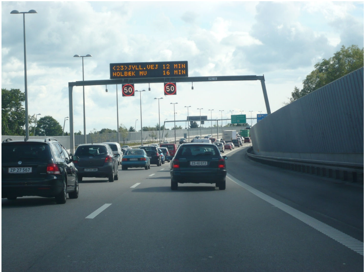
Figure 20: Speed control using variable message signs on Motorring 3 around Copenhagen
