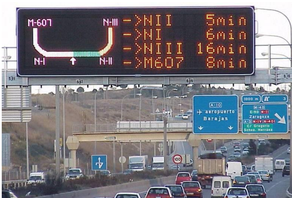
Figure 7:VMS on the A10 near Madrid in Spain
