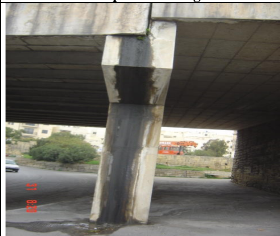
Deep Water infiltration on pier – Absence
