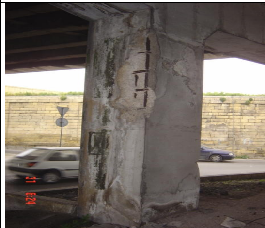
Important damage of concrete pier-
