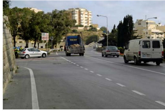
Short deceleration lane after tunnel [Junct EA13] Ghost splitter island, poor visibility left turn [Junct EA13]
