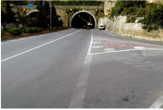
Short deceleration lane after tunnel [Junct EA13] Ghost splitter island, poor visibility left turn [Junct EA13]
