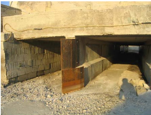
Inlet streamlined to reduce blockages
