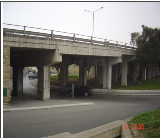
Elevation – RCI-Beams a Deck Slab Bridge – Absence of Neoprene bearings
