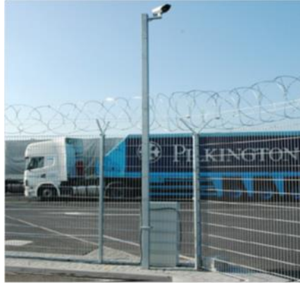
Figure 25: Fence and CCTV
