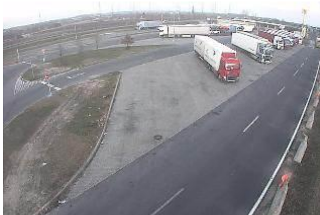
Figure 11: 3D picture of the TPA
