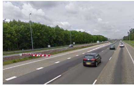
Figure 18: Entrance number nr. 3 with closed beam (median side). Tidal flow closed
