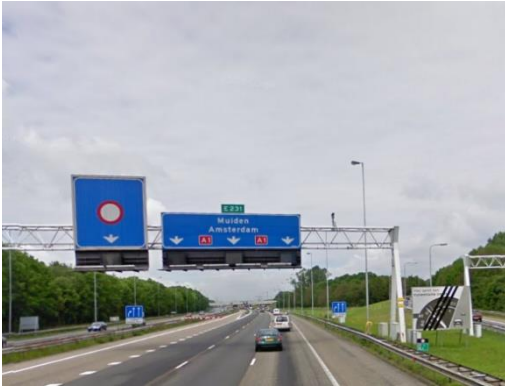
Figure 17: Entrance nr. 3 with dynamic route sign
