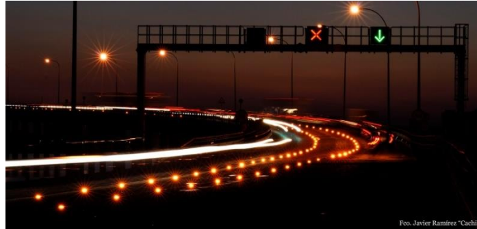
Figure 11: Image of the bridge
