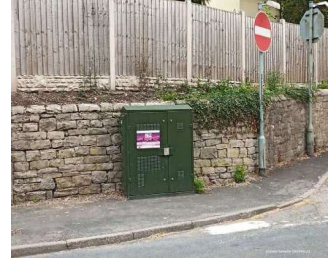
8.10 Example of feeder pillar / cabinet on footway, https://www.dovecomputers.com/
