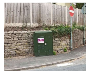
16.8 Example of feeder pillar / cabinet on footway, https://www.dovecomputers.com/
