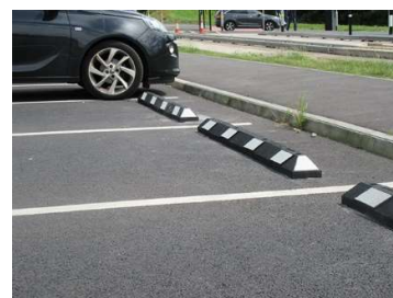
16.20 Examples of wheel stopper used in parking area, https://www.bollardstreet.com/
