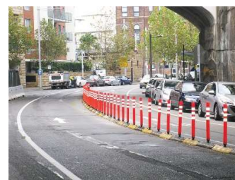
16.19 Examples of Collapsible delineator posts on carriageway, https://www.jaybro.com.au/
