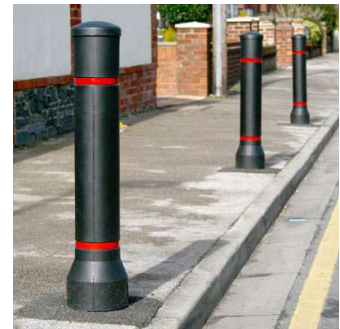
16.4 Example Metal Bollards with retroreflective strip, https://gil.glasdon.com/
