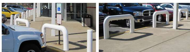
16.6 Example of metal barriers used to delineate footway, https://www.innoplast.com/
