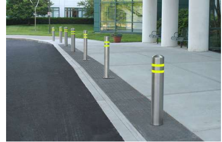
16.3 Example of Stainless-Steel Bollards when used on footways, https://www.indiamart.com/
