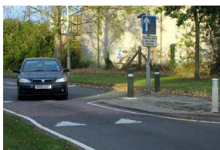
Figure 17: Road narrowing with road hump
