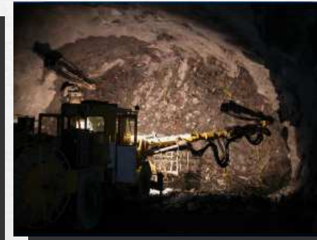
Drill and Blast
